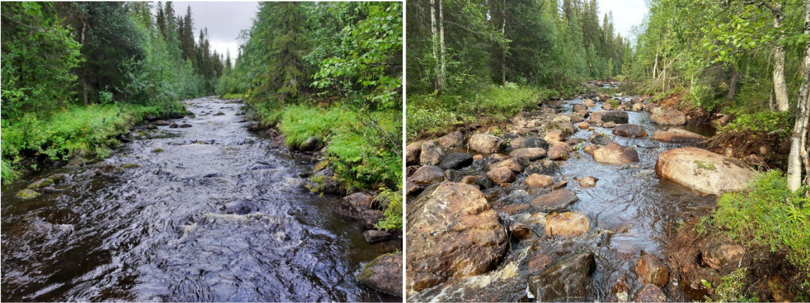
Figure 3 Before and after restoration in Vargån, Västernorrland
