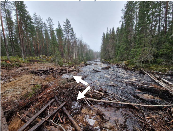
Figure 8. Two dead wooden debris sites along the outer bend of a restored river stretch. The logs are positioned in a gradient up the river bank, to ensure the logs get different amount of water coverage during floodings.
