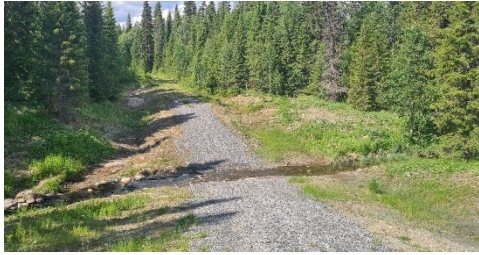
Figure 12. Total removal of barrier JC5_093. Executer: Billerud
