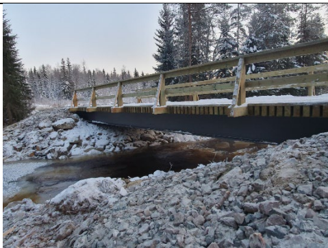
Figure 14. Bridge. Executer: CABVn
